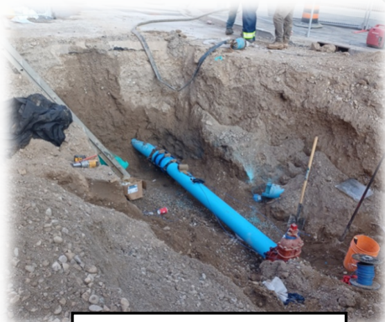
Example of Watermain connection to existing watermain
